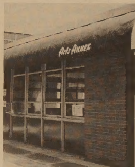
What was once the Maintenance Building (on what was once the edge of the campus) is now the Arts Annex, providing new spaces for the college's music and art programs.
