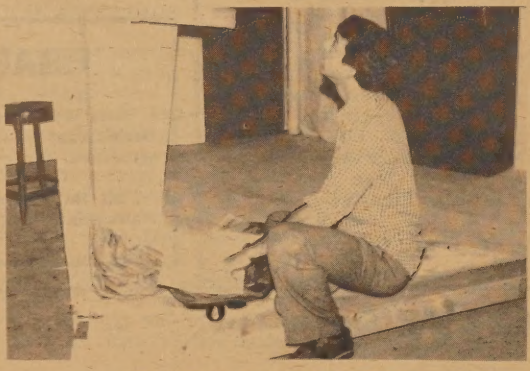
Tom Mangino - Checking Set Construction.
