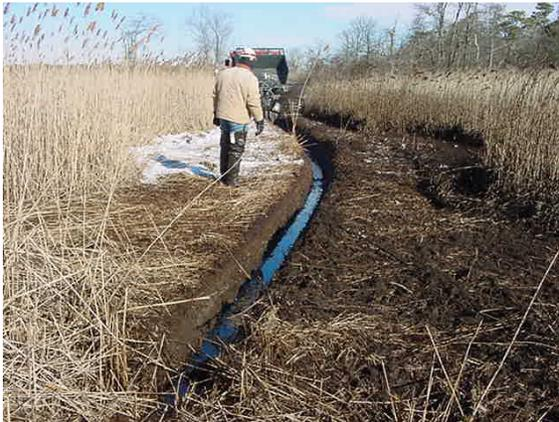
Figure 5 - Pisten Bully creating tidal channel along landward side of Area 1. In order to mitigate potential spreading of *Phragmites*, the soil from tidal channel along this portion of the marsh was deposited upland into an existing *Phragmites* stand. Environmental monitor in foreground.
