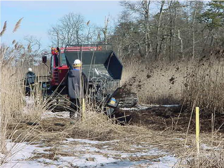
Figure 11 - Monitor watching Pisten Bully cutting tidal channel in Area 1 to ensure track follows markers.
